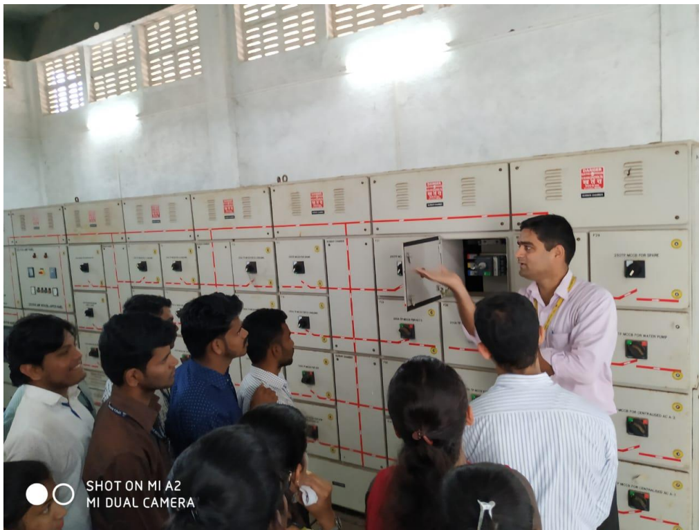
Near main Power control center.
